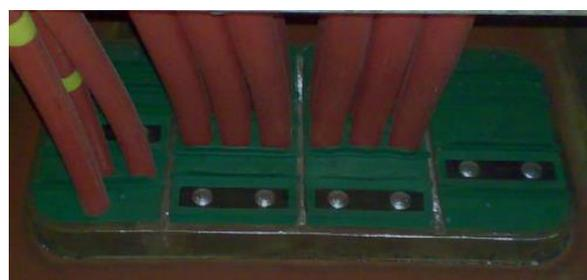
Figure 2: A view of a correctly installed seal packing system.
